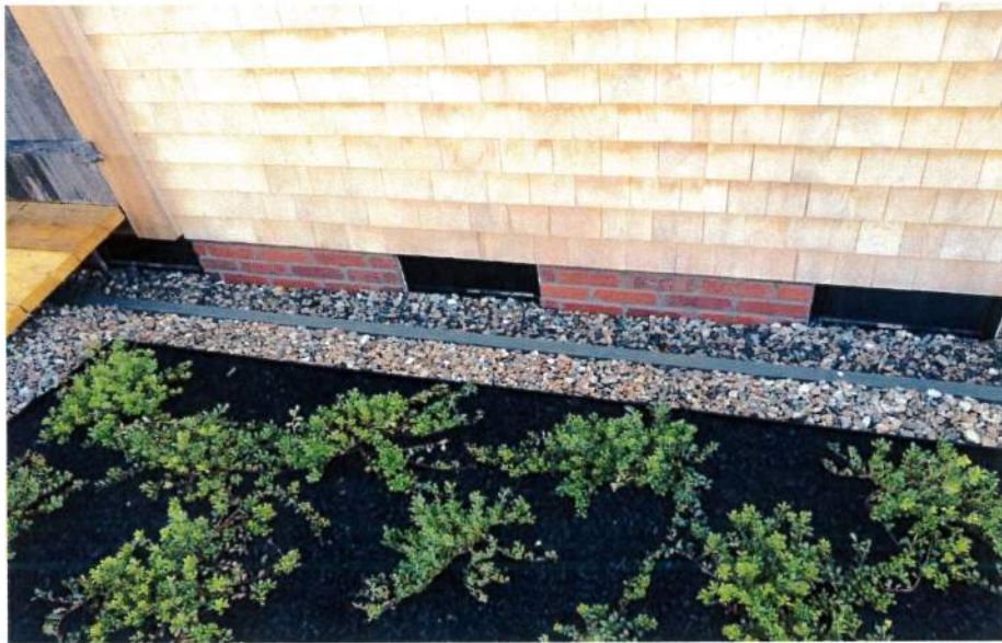
West Side, Flood Openings
