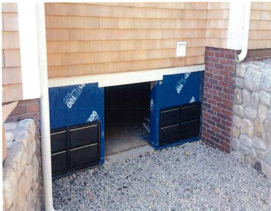
East Side, Flood Openings
