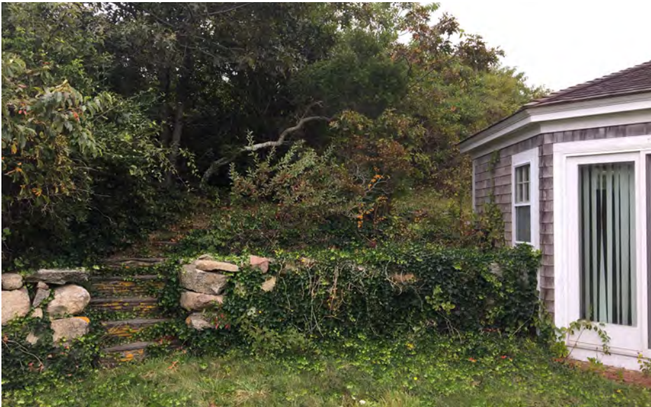
View of north side of the house, lawn historic garden walls and a mix of invasive and native vegetation.
