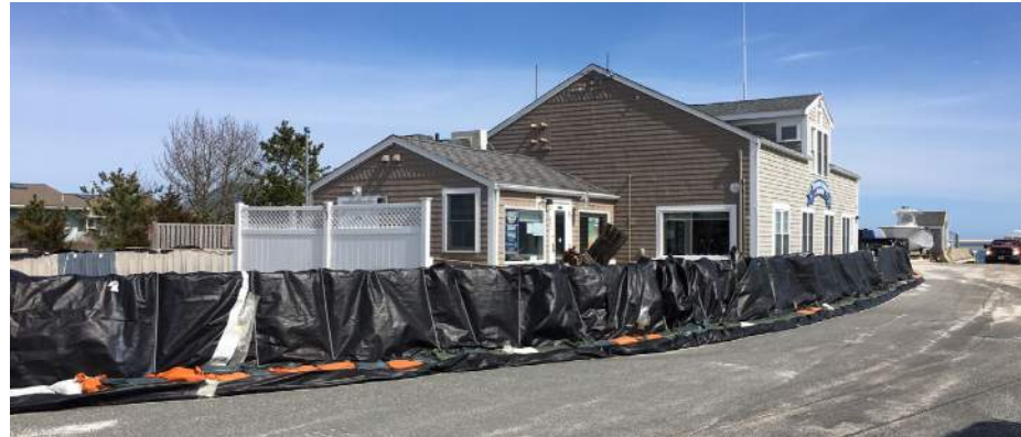
Temporary barrier deployed at Chatham Outermost Harbor Marine.
