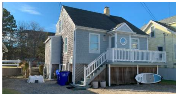
Small side addition to house mechanical equipment in an elevated interior space.
