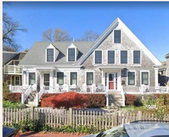
Historic buildings in Wellfleet and Provincetown with narrow elevated front decks and streetscape plantings that provide a gradual transition to the higher entry elevation.
