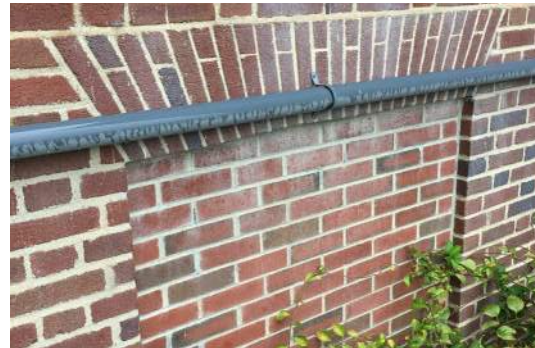
The original location and size of a basement window is preserved with inset bricks.
