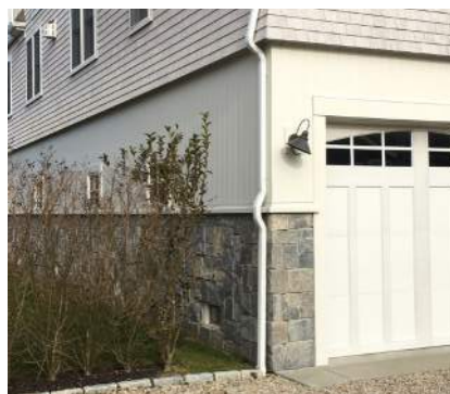
Stone facing provides a flood resistant material on wall sections that are likely to be exposed to flooding.
