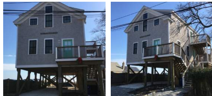
This building was originally set at the street edge but was pulled back about 10 feet to soften the impact of elevating it approximately 11 feet above its original height. The change still has a dramatic effect on the district's character.
