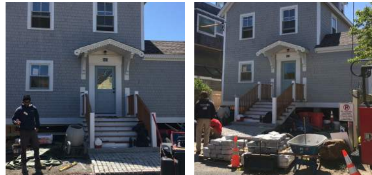
This historic structure was elevated four feet, less than would be required for a non-historic structure, in an effort to preserve the historic streetscape.
