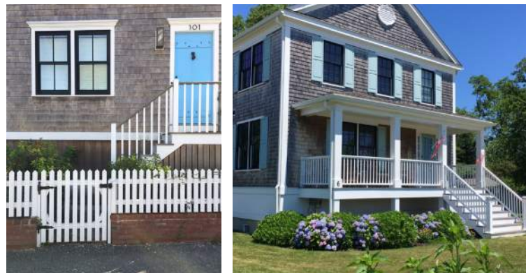
Fencing, plantings, porch details, and trim should reflect the established neighborhood character.
