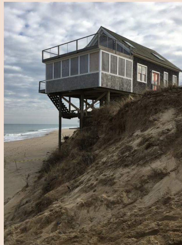
This Truro building and another next door were relocated farther inland to move them away from the eroding coastal bank and flood hazard areas.
