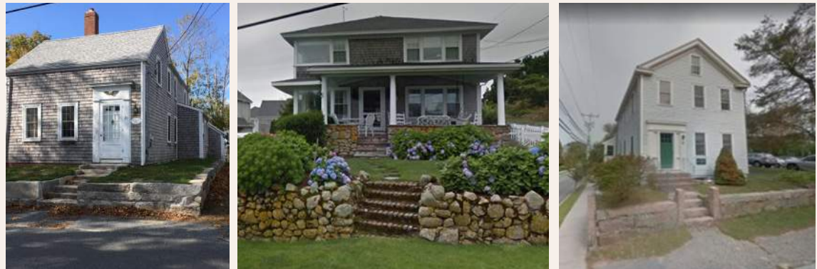
Historic buildings in Sandwich, Hyannis Port, and Woods Hole on sites elevated with low stone walls.
