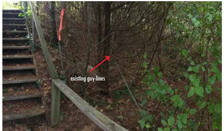
View of slope looking northeast where previously installed guy-lines have girdled white pine trees.
