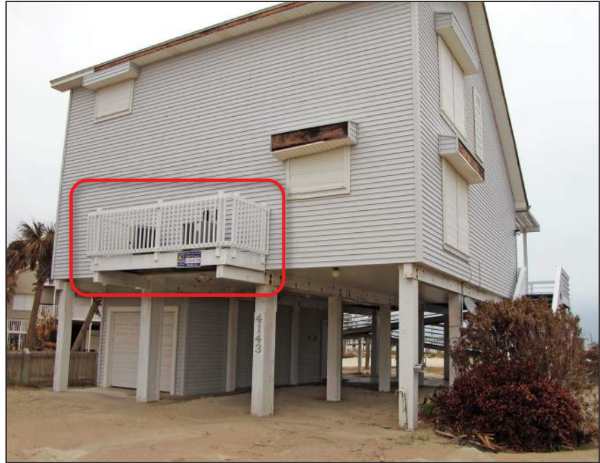
Figure 4-2. Elevated HVAC condenser units in a coastal zone with a protective railing installed (Galveston Island, Texas).
