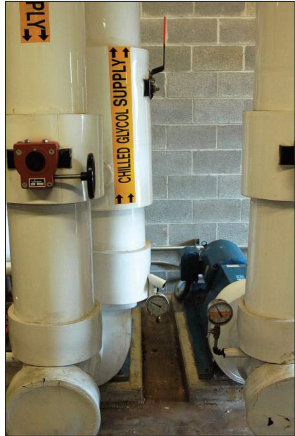
Figure 5-4. Chilled water pump, Georgetown, Delaware.
